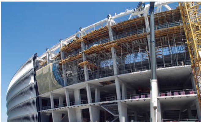
▶ Safe construction of cantilever slabs
