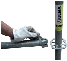
1.- Hook in the horizontal ledger
