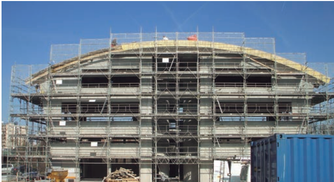
▶ Roof-edge protection work on the roof edge
