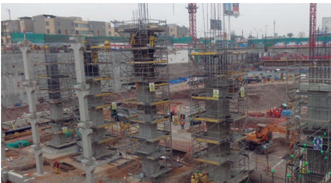
► Scaffold towers in column construction
