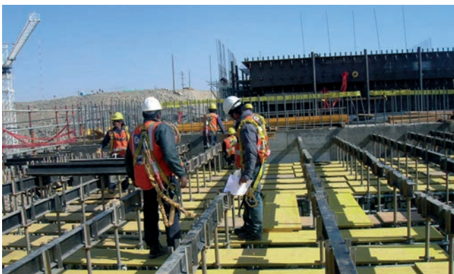
▶ Safe falsework assembly
