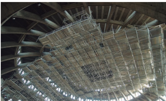
▶ Suspended working platform to work under the roof
