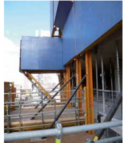
Each panel consists of two vertical MK-180 walers (masts) to which all components are assembled and which guide the structure.
