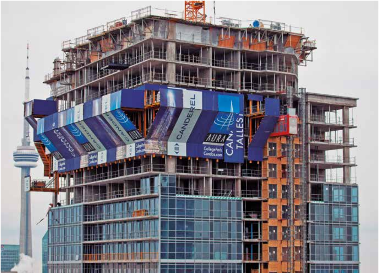
■ The HWS Hydraulic Windshield System protects the perimeter against adverse weather conditions and prevents objects from falling from higher levels. Moreover, different HWS structures enable the storage of material around the perimeter of the building, and thus minimise the use of the crane.
