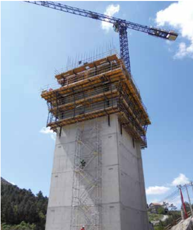
ATR self-climbing system and BRIO scaffolding access stair in pier construction
