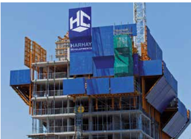
Outside formwork hanging from the upper MK structure of the ATR system
