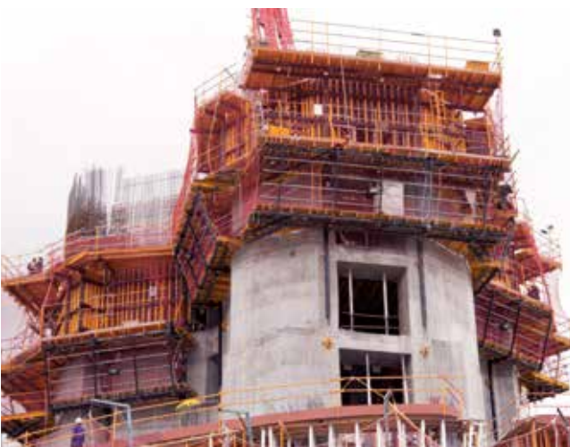
ULMA engineers adapted the formwork to the 4 different shaft sections.
