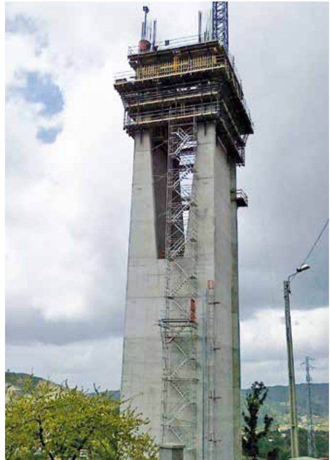
ATR self-climbing system and BRIO scaffolding access stair in pier construction
