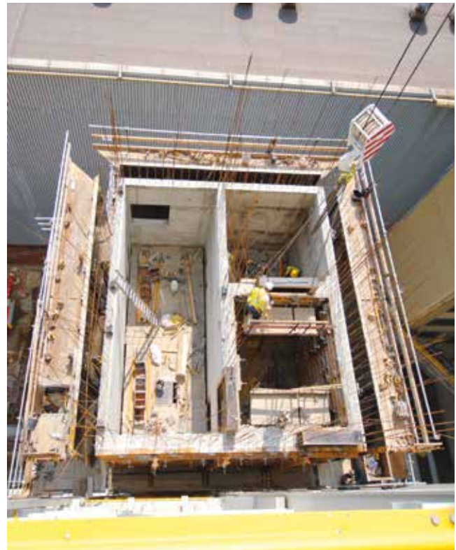
The solution for the limited space between the lift shaft and the steel structure of the building with ATR self-climbing system, two KSP shaft platforms and HWS system with formwork.
