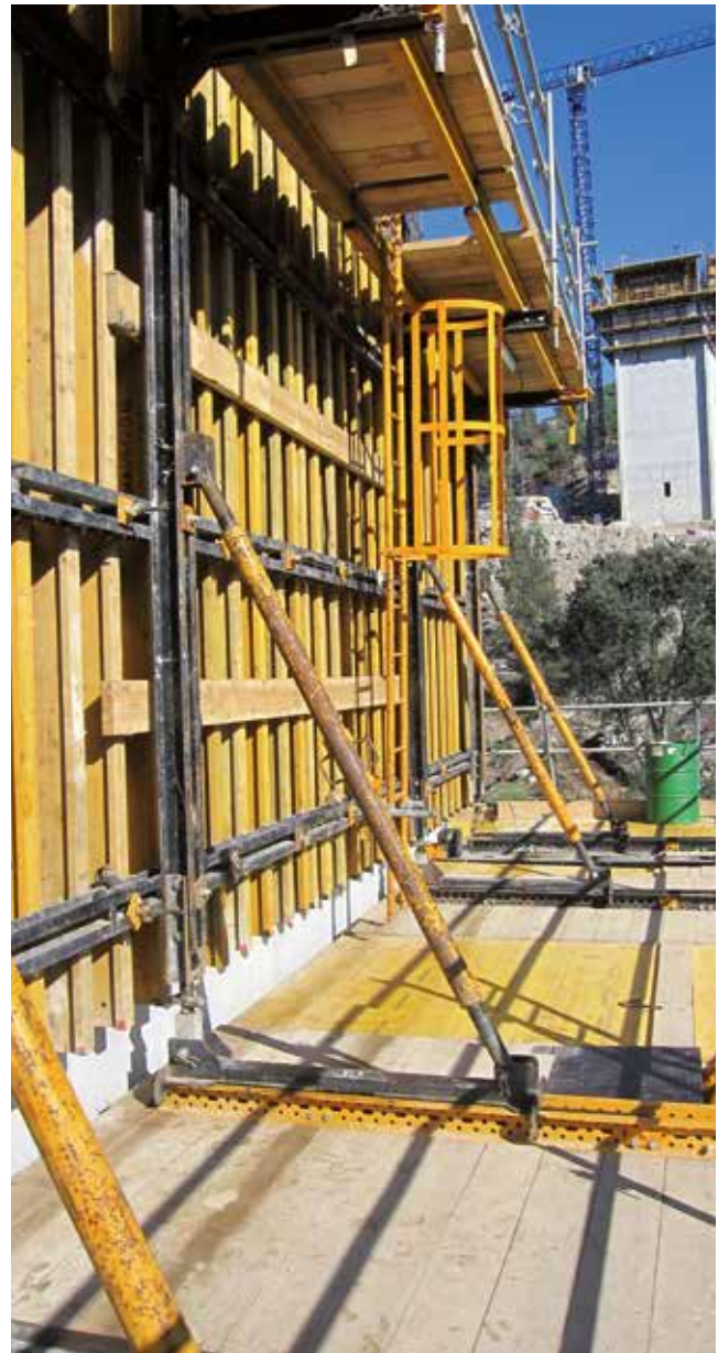
Formwork adjustment and plumbing system with stripping system of up to 70 cm
