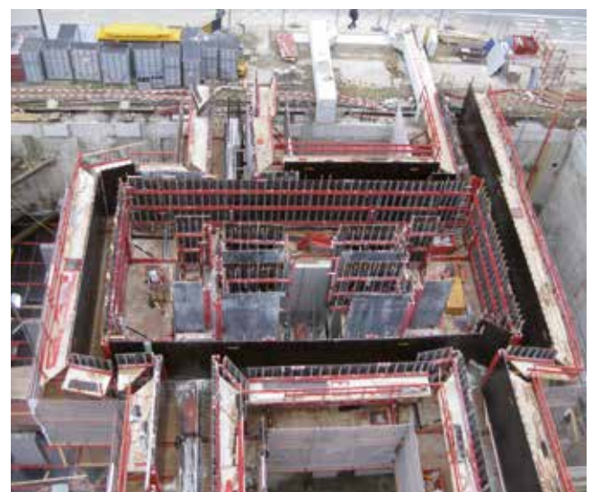
12 m long platforms with narrow platform solutions for inside
