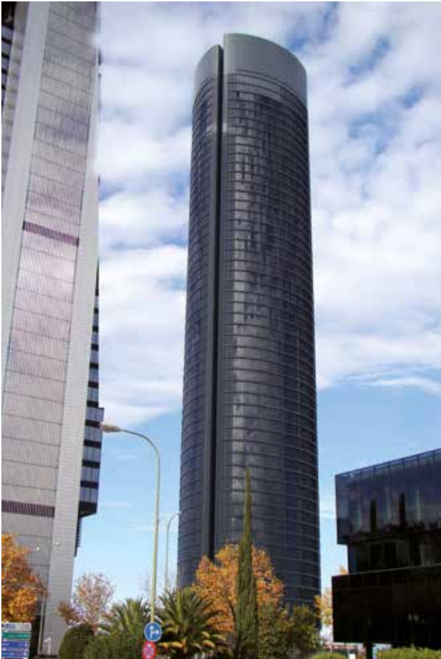
A five star luxury hotel with 500 rooms occupies the first 33 floors while the rest are offices.
