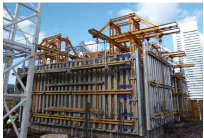
Outside formwork hanging from the upper MK structure of the ATR system
