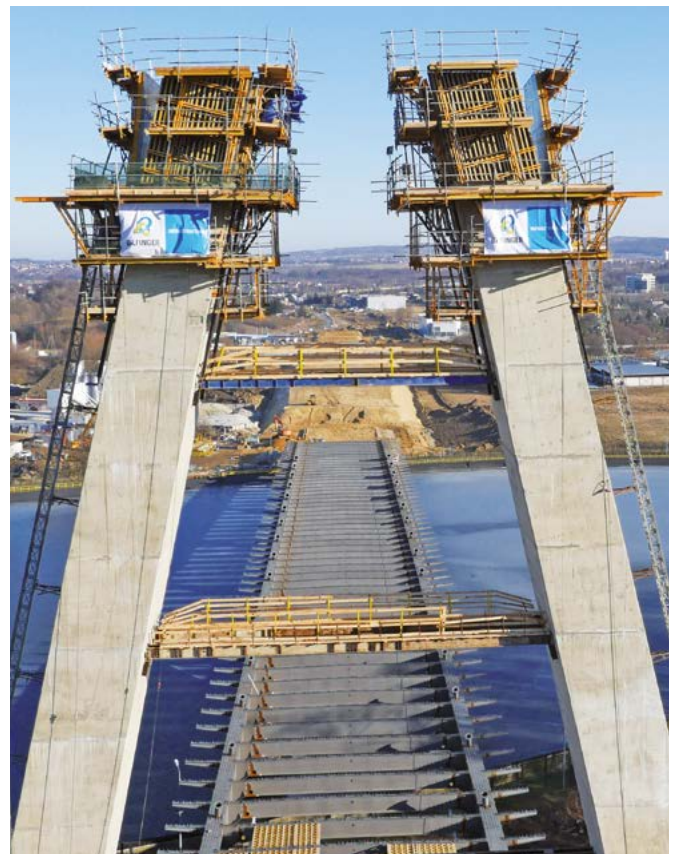
▶ ATR used in inclined pylon construction
