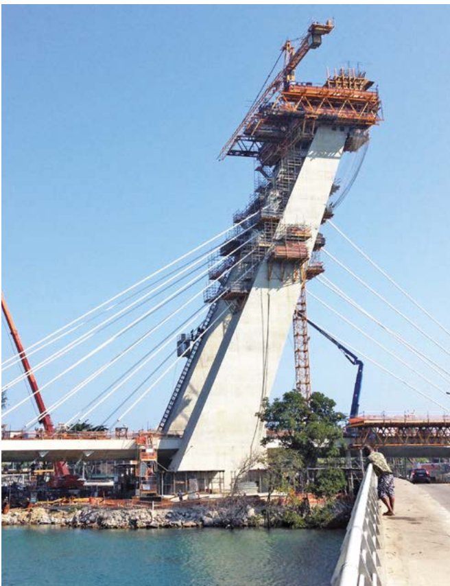
▶ ATR used in inclined pylon construction
