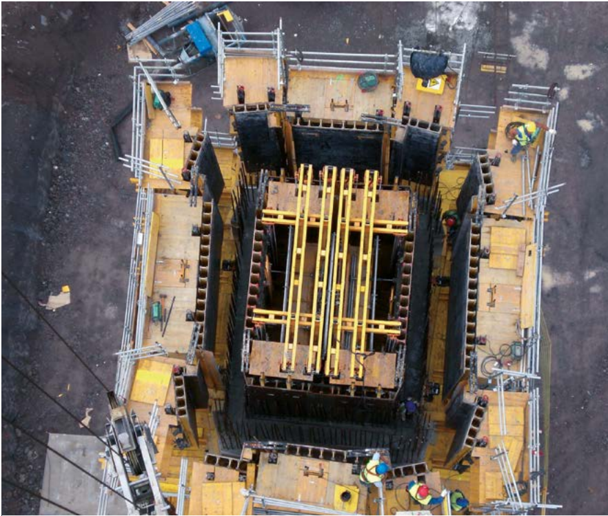
▶ Exterior and interior formwork free from interferences above
