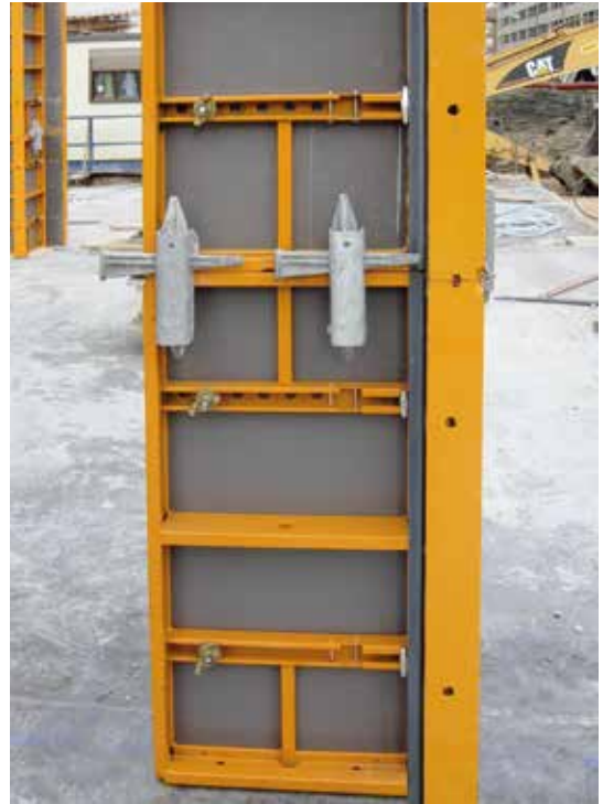
Panels join with two clamps
