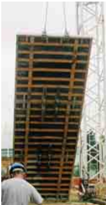
▲ These pieces provide rigidity and stability in hoisting
