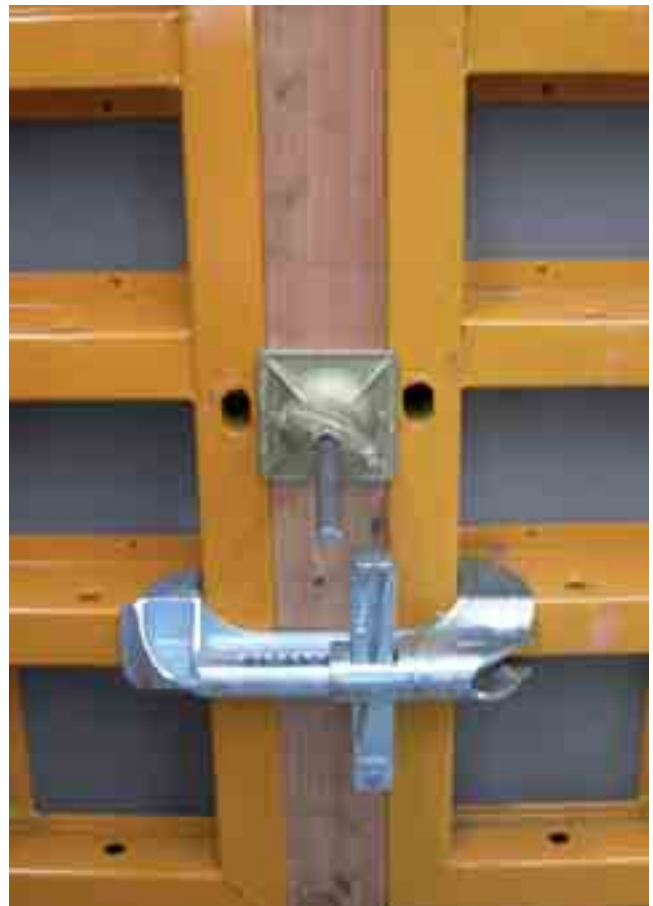
▲ This clamp can cover fillers between panels up to 10cm wide
