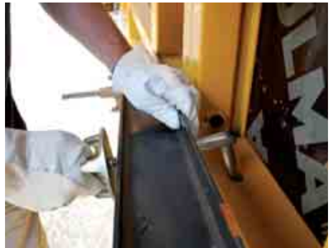
▲ Anchor of the Waler Hook in ORMA's Panel
