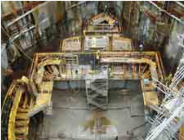
▲ The ORMA Modular Formwork system is capable of providing solutions for different geometries encountered when erecting vertical structures
