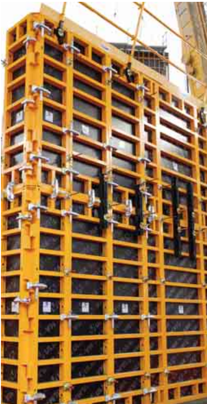
▲ The clamp joins panels in the edge
