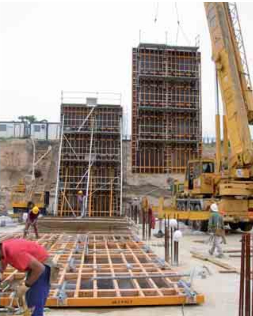
▲ Lifting gangs including working platform in different levels
