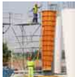
CLR Circular Column Formwork Circular column formwork, designed to solve the different column diameters easily
