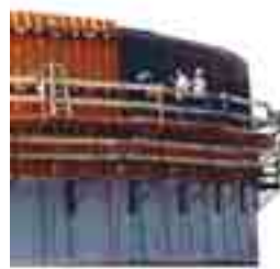
Circular Sheet Formwork BIRA Formwork system designed for circular wall configurations
