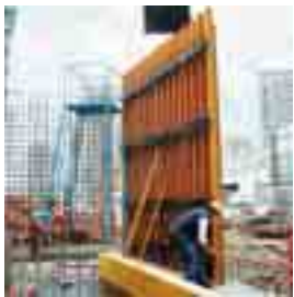
ENKOFORM V-100 Bracing System Wall and Column Formwork with Steel Walers and Timber Beams
