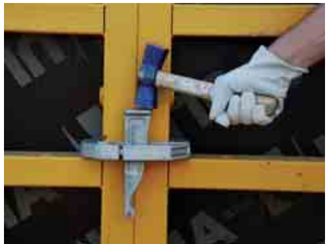
▲ The clamp joins panels in the edge
