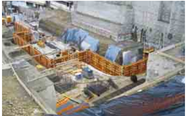
▲ The ORMA Modular Formwork system is capable of providing solutions for different geometries encountered when erecting vertical structures
