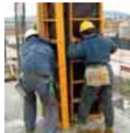
LGR Column Formwork Column formwork using light panels
