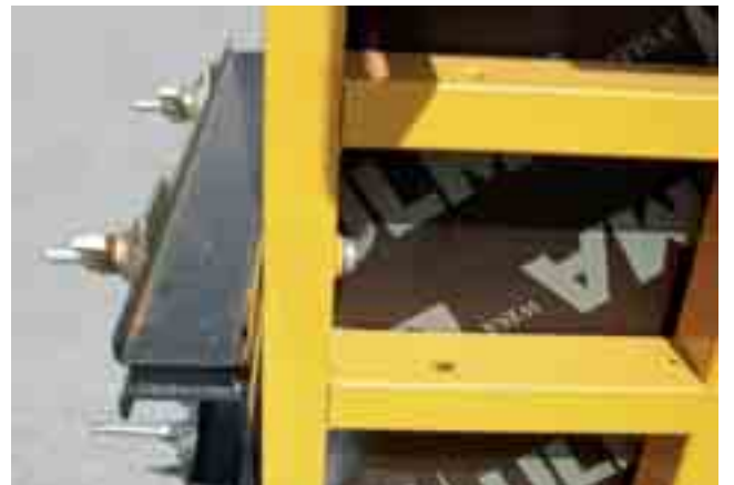
▲ Fixing the Waler to the panel using Universal Panel Bolt
