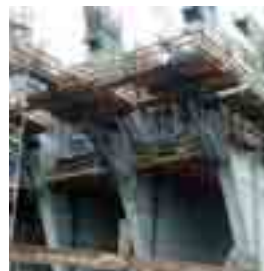
Formwork Climbing Systems Climbing and self-climbing systems for any height
