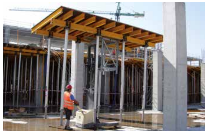
► VR Table pre-assembled slab formwork with VM-20 beam
