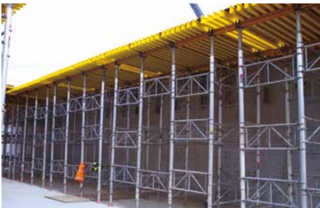
► VR Table pre-assembled slab formwork with MK waler
