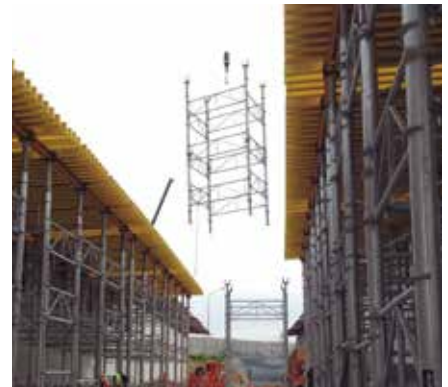
▶ ALUPROP tower lifting
