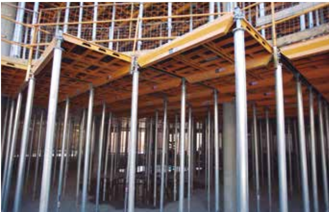
▶ CC-4 aluminium slab formwork
