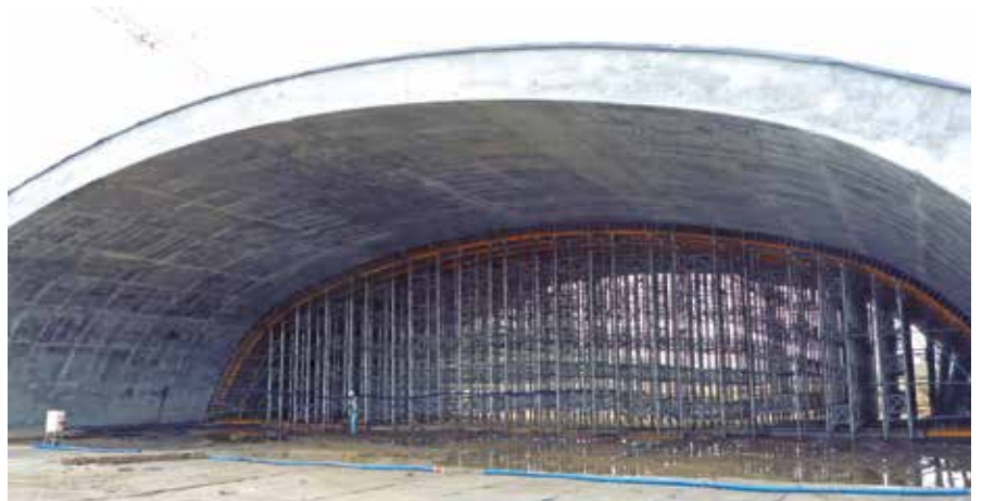
▶ Shoring in cut-and-cover tunnels
