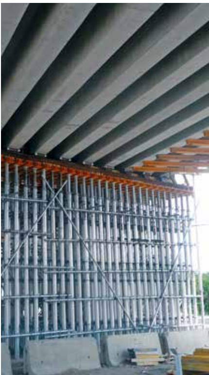
▶ Shoring in bridges
