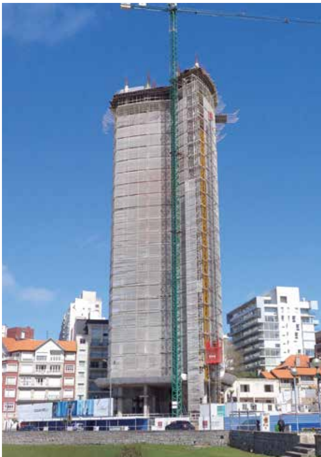
► Laying slabs with an irregular geometry
