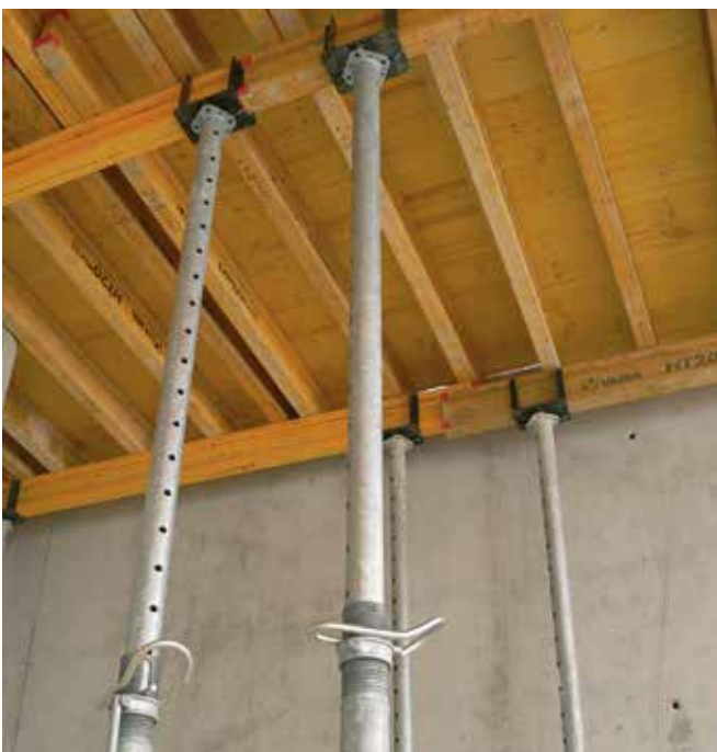
► Formwork against a single wall with overlapping beams
