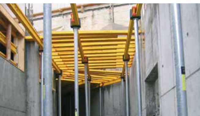
► Formwork against a single wall with overlapping beams
