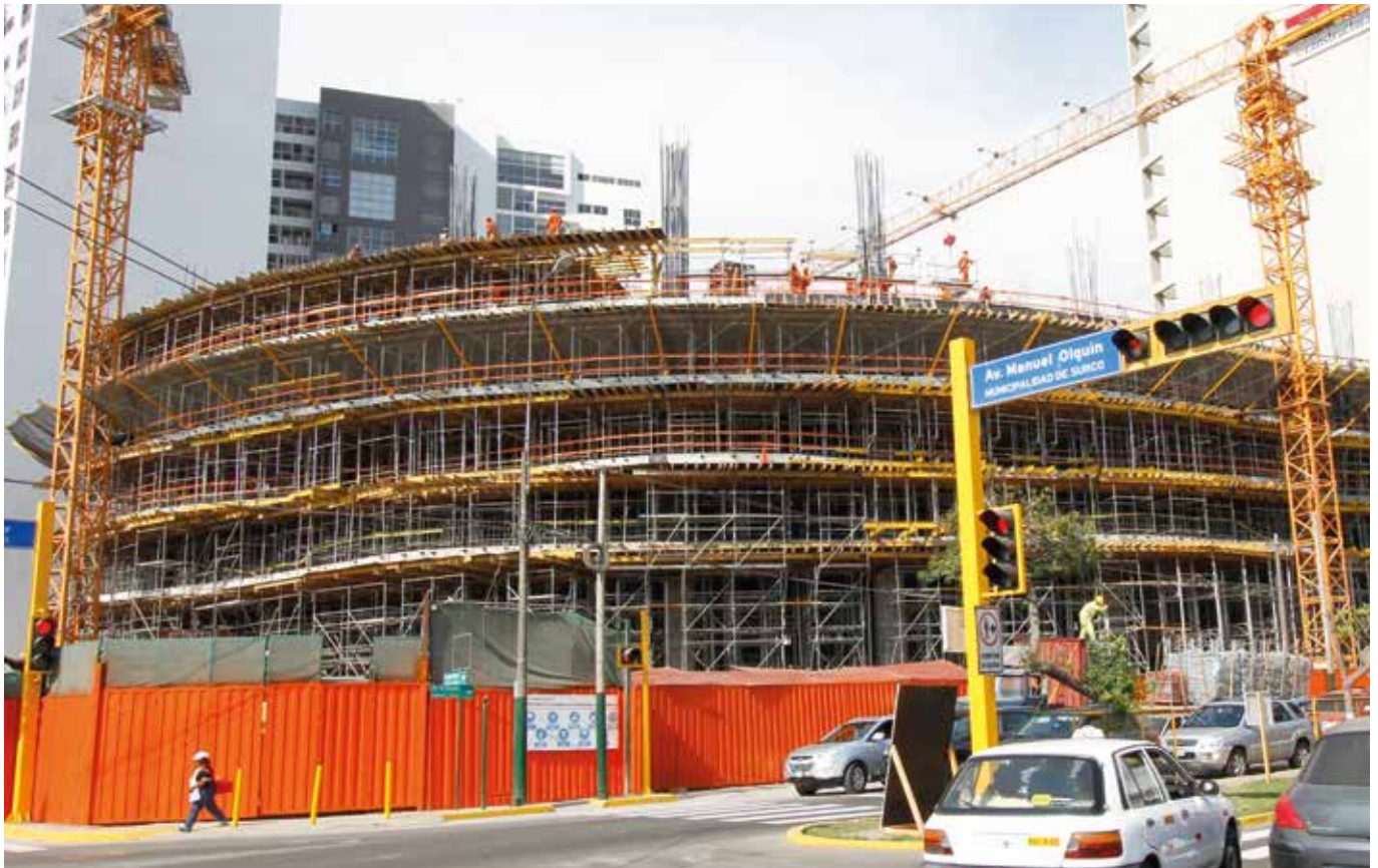
► Slabs laid with vertical ENKOFLEX with steel props, aluminium towers and falsework
