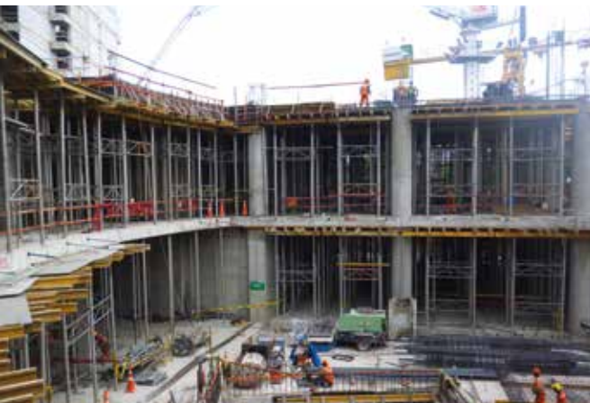
► Shoring of large loads with ALUPROP towers
