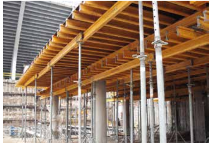
► Wooden beams at different levels
