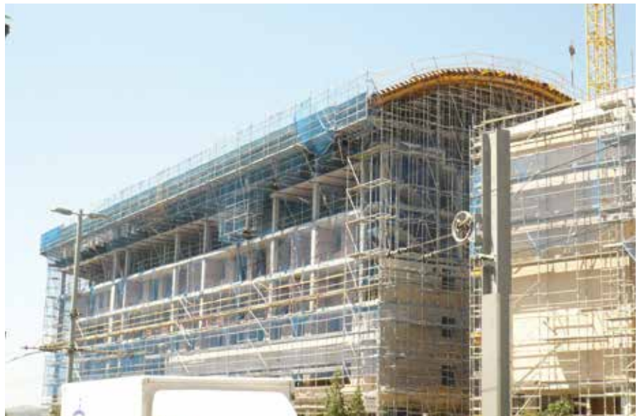
► Inclined surface with ENKOFLEX on the falsework
