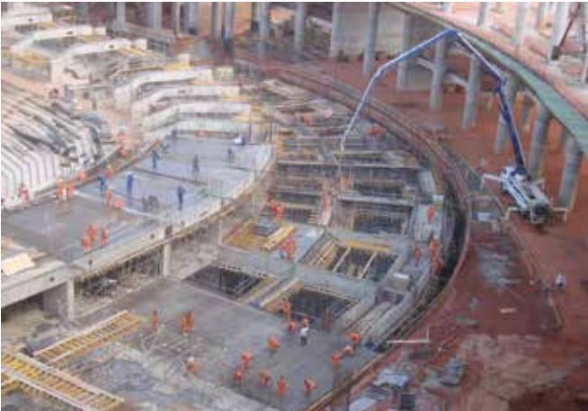
► Construction of intermediate and perimeter drop beams
