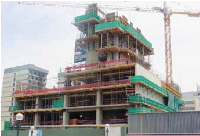
► Shoring with certified EP steel prop
