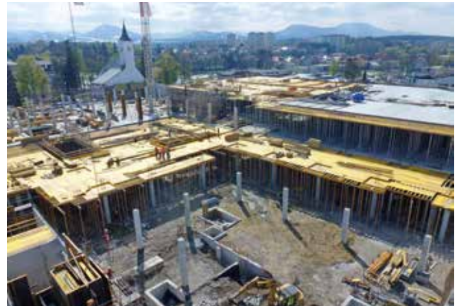
► Shoring with SP prop
