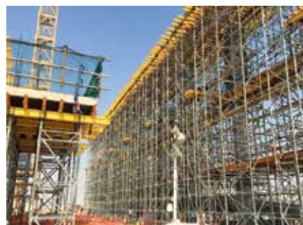
► Shoring at a height with T-60 falsework
