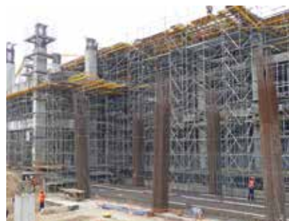
► Stable shoring with BRIO falsework
