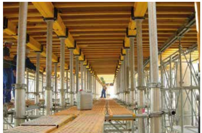
► Formwork assembly platforms on falsework tower
