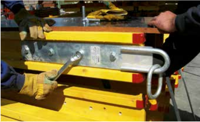
► Placing the lifting bracket on the beam web
