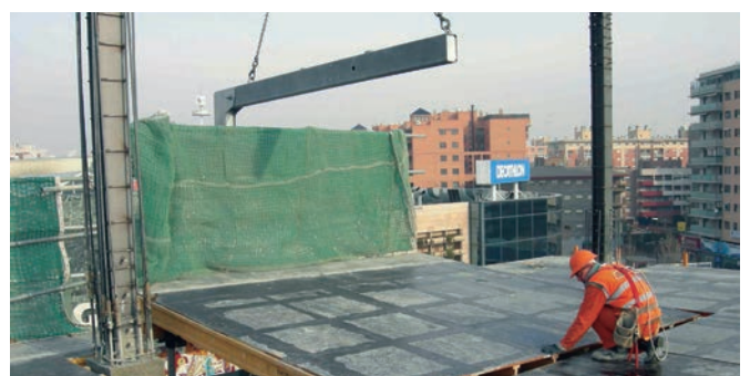
▶ Lifting and installation of tables with attached handrails
