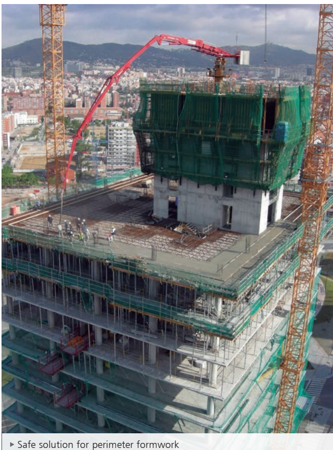
▶ Lifting and installation of tables with attached handrails
