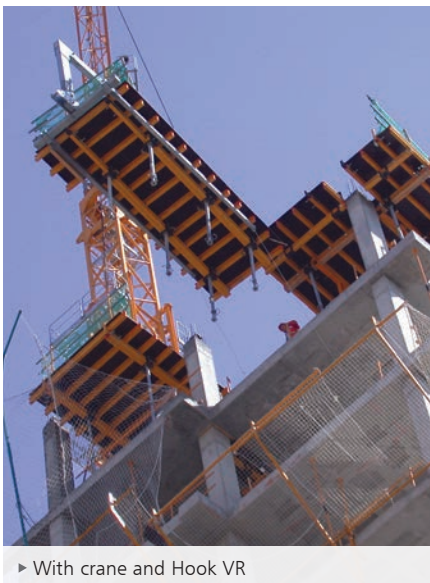
► With crane using VR compensator
