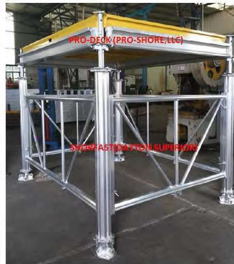
Perfect Compatibility of SHORFAST(as shoring)and PRO-DECK (as decking form)
