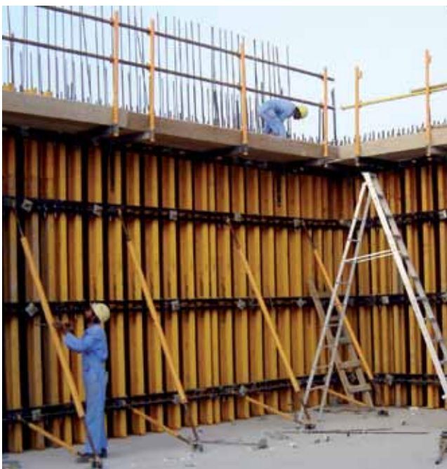
▲ VM-20 beams in ENKOFORM V-100 vertical formwork ▲
