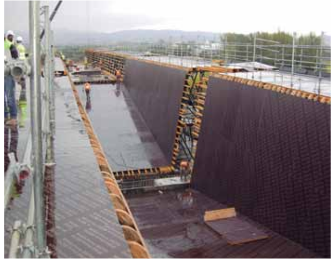
▲ Phenolic plywood as shuttering face in ENKOFORM H-120 formwork of a viaduct under construction
