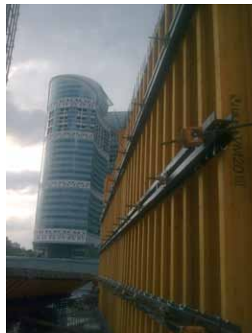
▲ VM-20 beams in ENKOFORM V-100 vertical formwork ▲
