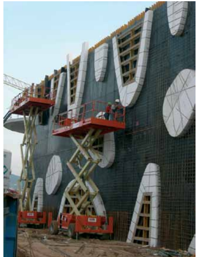
▲ High-quality finish of fair-faced concrete walls with phenolic plywood in ENKOFORM V-100 vertical formwork
