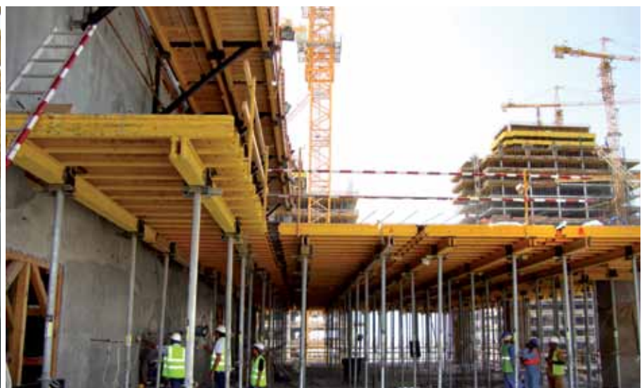
▲ VM-20 beams in Table VR horizontal formwork and for working platforms on climbing brackets
