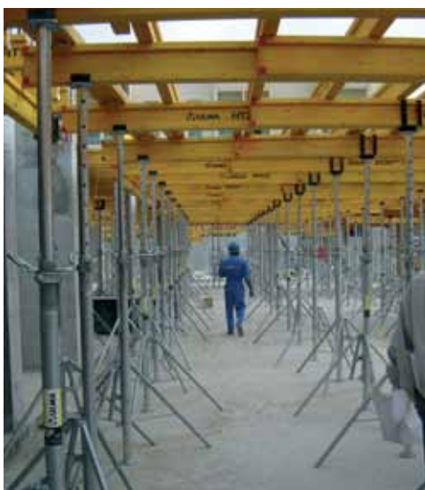
▲ VM-20 beams in ENKOFLEX horizontal formwork
