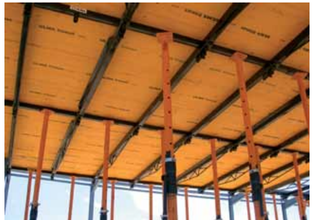
▲ 3-layer board Trimax in RAPID horizontal formwork ▲
